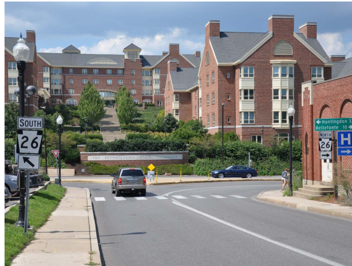
Left: The intersection of College Avenue and High Street is especially hazardous for pedestrians due to the free flow traffic lanes and the absence of crosswalks over College Ave.
